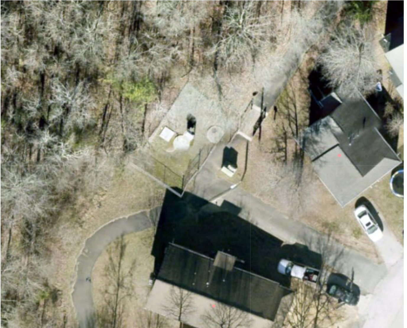
Nassaw Lift Station.
