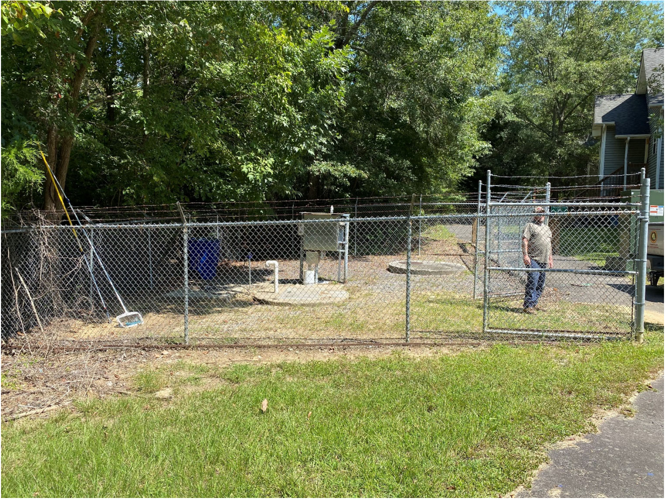
Nassaw Lift Station.
