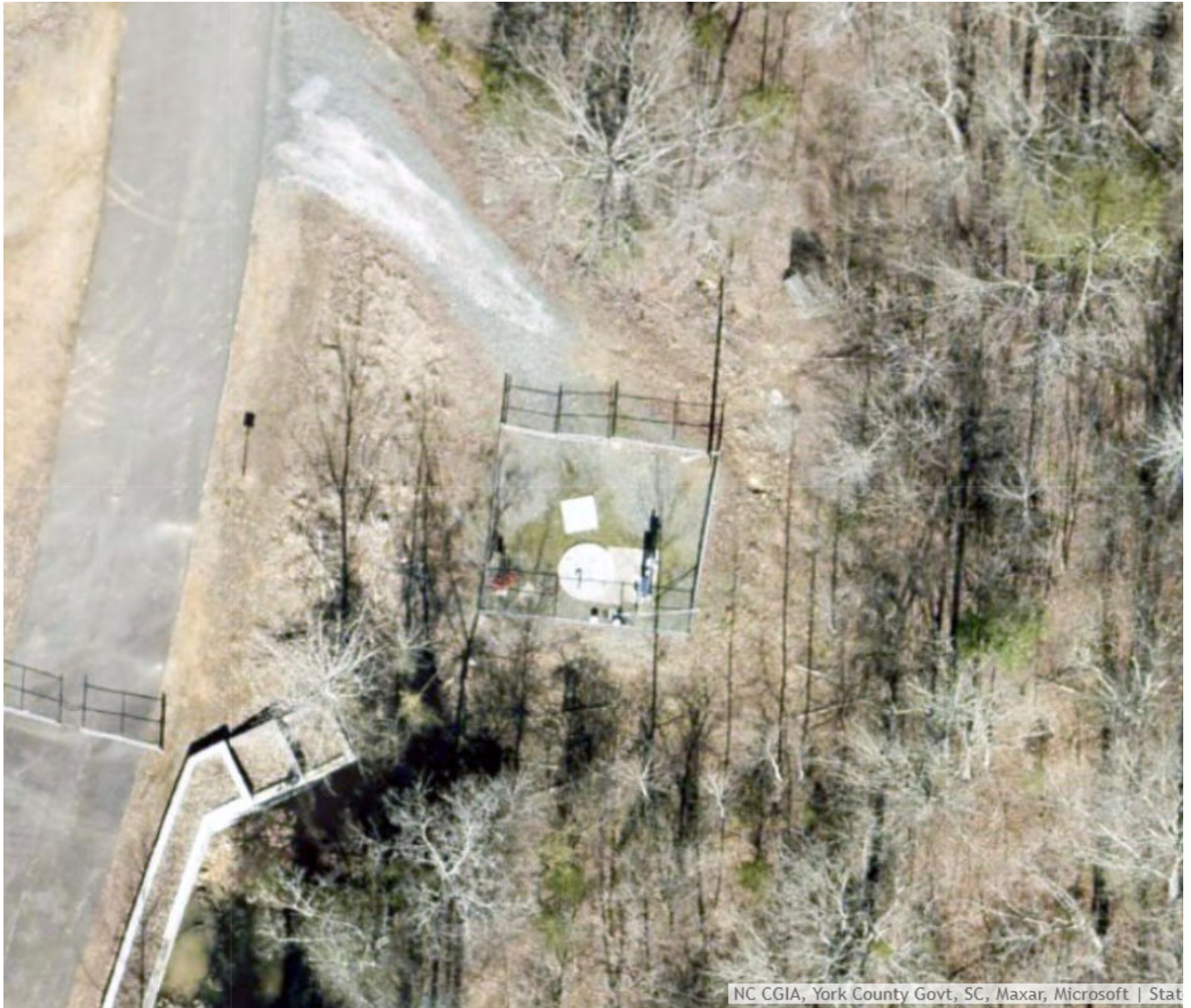
Sturgis Lift Station.
